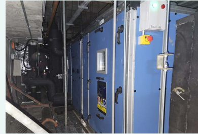
Replacement of AHU
